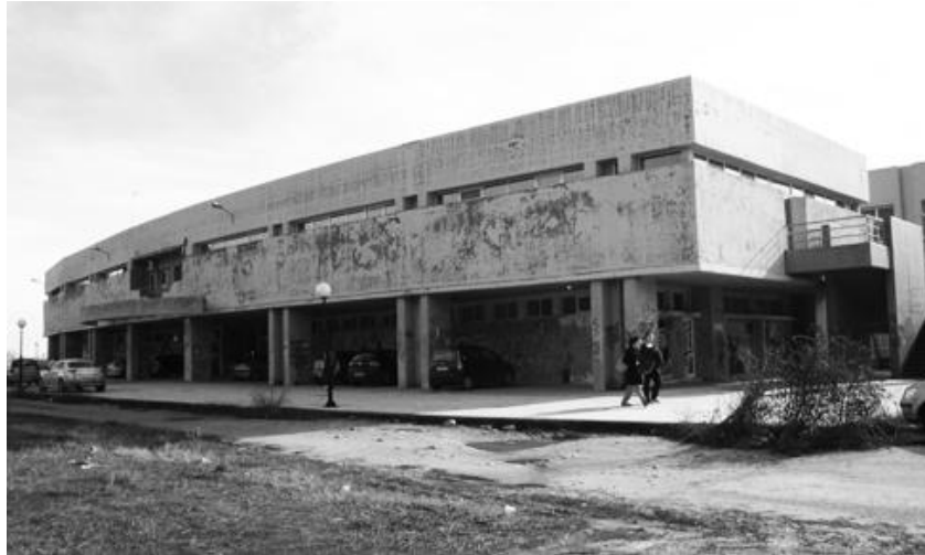
Figure 1. The northern façade of the building.
